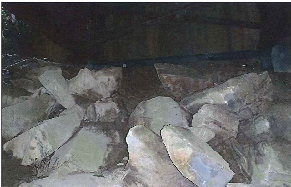
CK2368 Left Abutment
