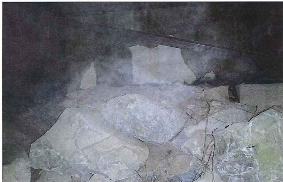
CK2368 Right Abutment
