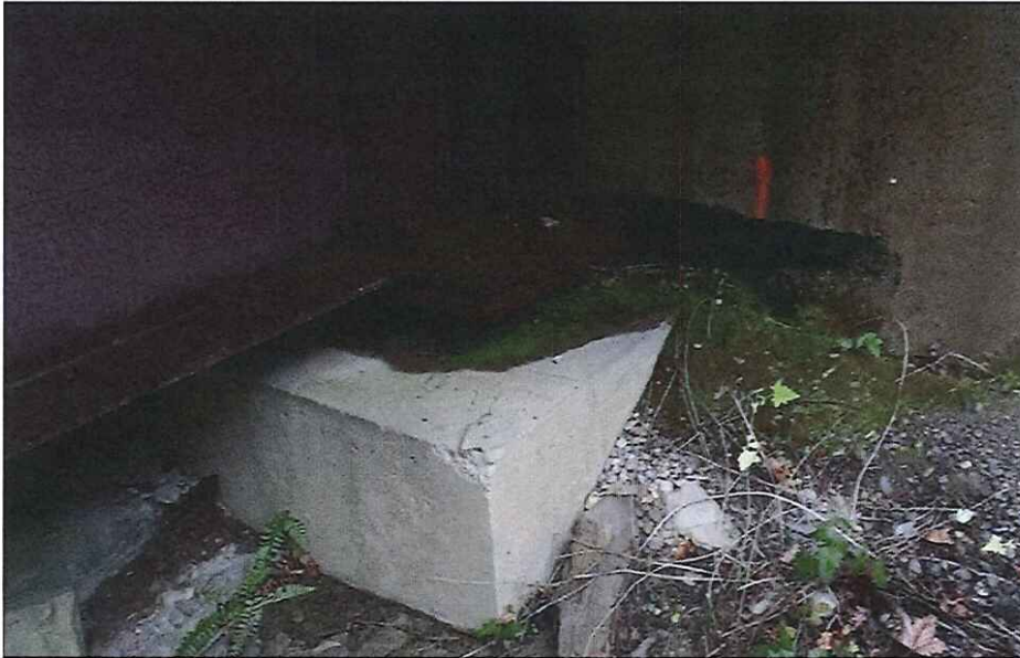
CK2368 Right Abutment Bearing
